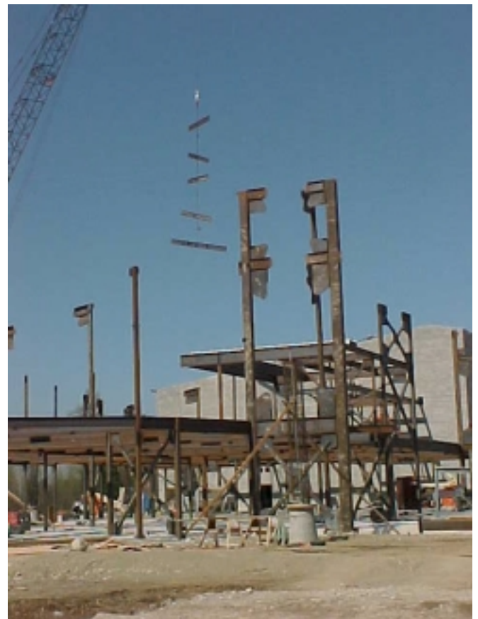
Area B Structural Steel Erection, 2 nd Floor.
