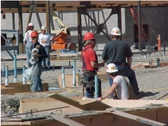
John Carlson, Jeff White, Robert Clark, and Bob Fisher setting up Area C slab pour at Job 697 – New Bethel H.S. #3.
