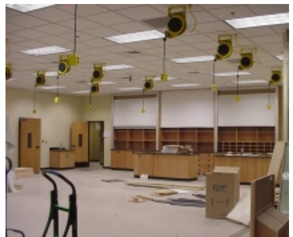
Art, Sculpture, etc. classrooms all have power available for each work station from the ceiling.
