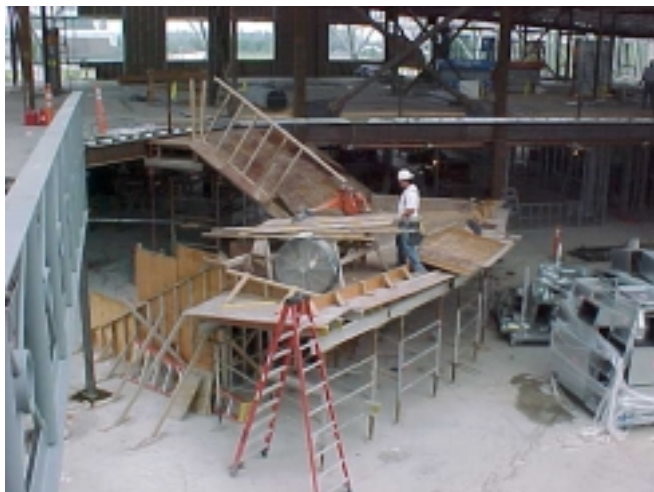
This photo taken on 06/22/04 shows Kidder Anderson and Brian Michalek forming the main stair at the Commons.
