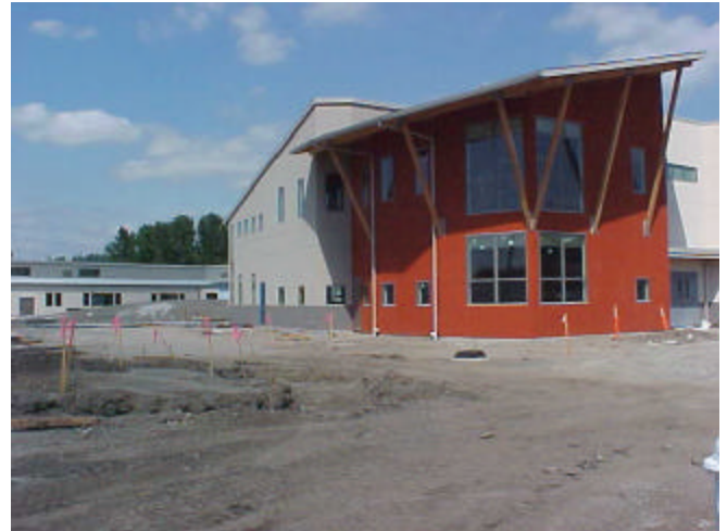
Bldg. A in Foreground, Building C in Background 06/29/05
