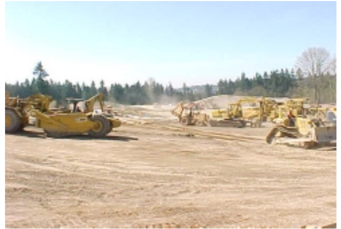
Forming retaining wall footings, 04/09/02
