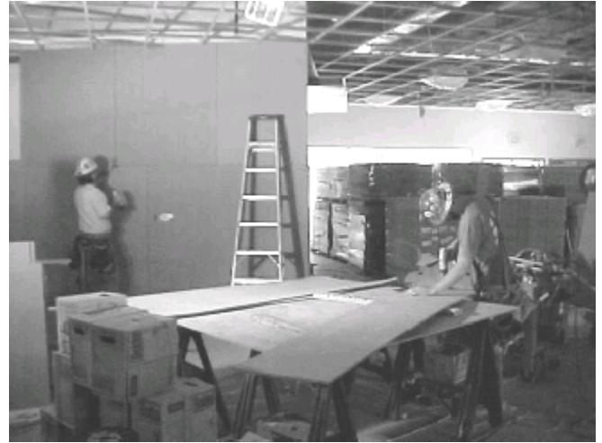
Installing MDF Board
