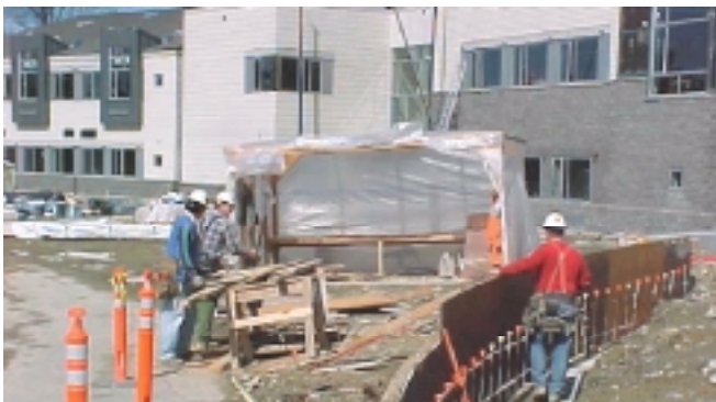
Forming Retaining Walls
