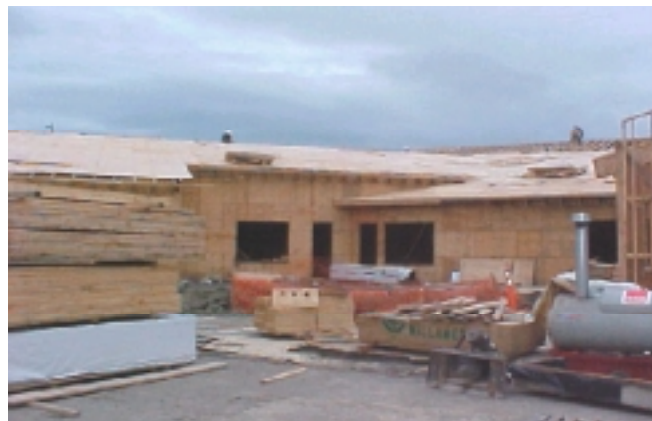
Construction of LaVenture Middle School's New Wing, well underway, 04/08/03.
